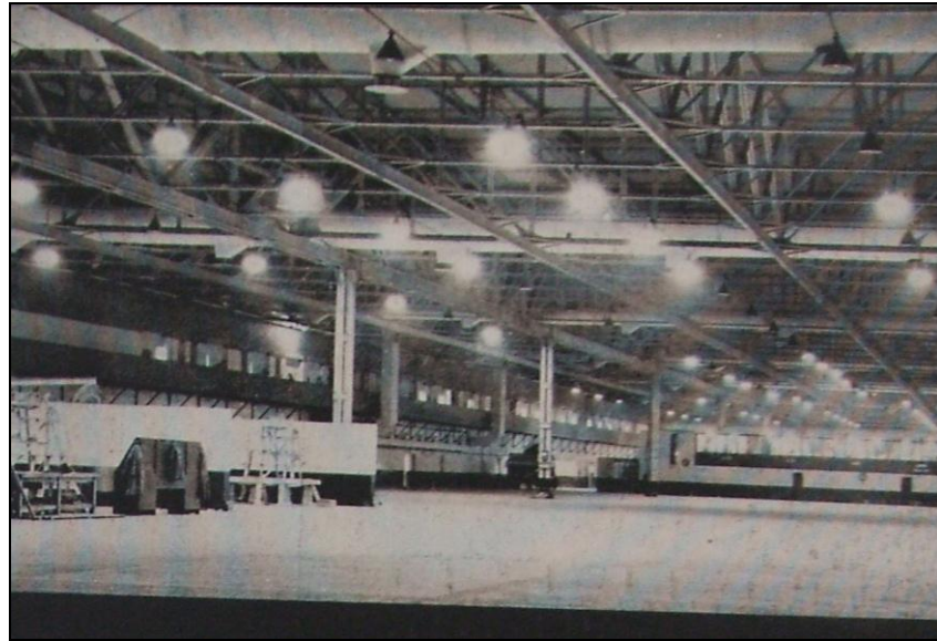
Plate 8.19: Plans for a buried Factory Type H (top left and right); Photograph of the appearance inside a buried factory (bottom).
