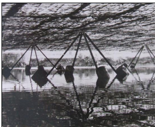
Plate 7.23: Photographs showing the arrangement of 'Table' (left) and 'Pyramidal' (right) floating supports.
