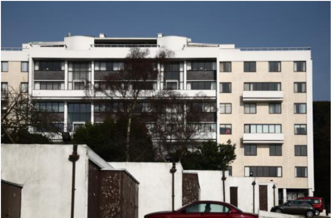
Fig. 5.2: Highpoint Two (photograph by Steve Cadman).
