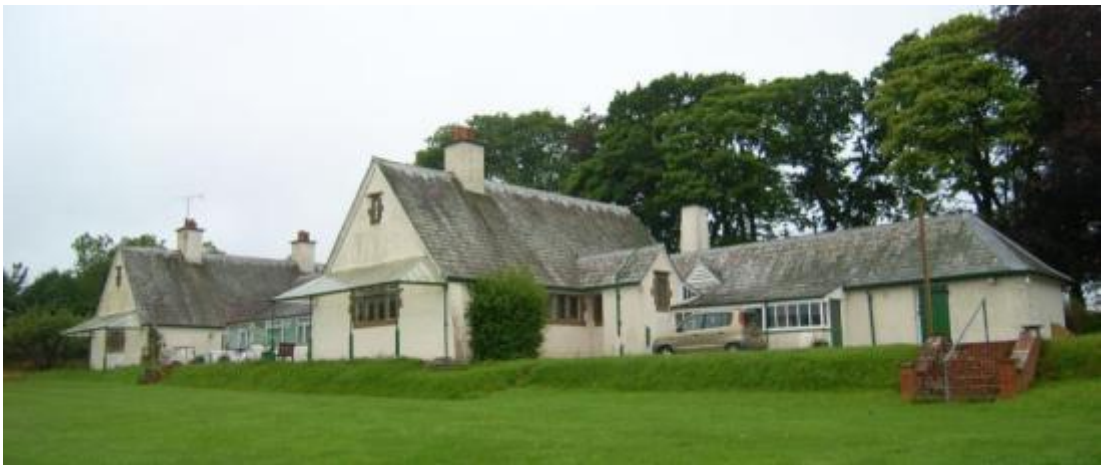
Fig. 3.3: Winsford Cottage Hospital (rear elevation).
