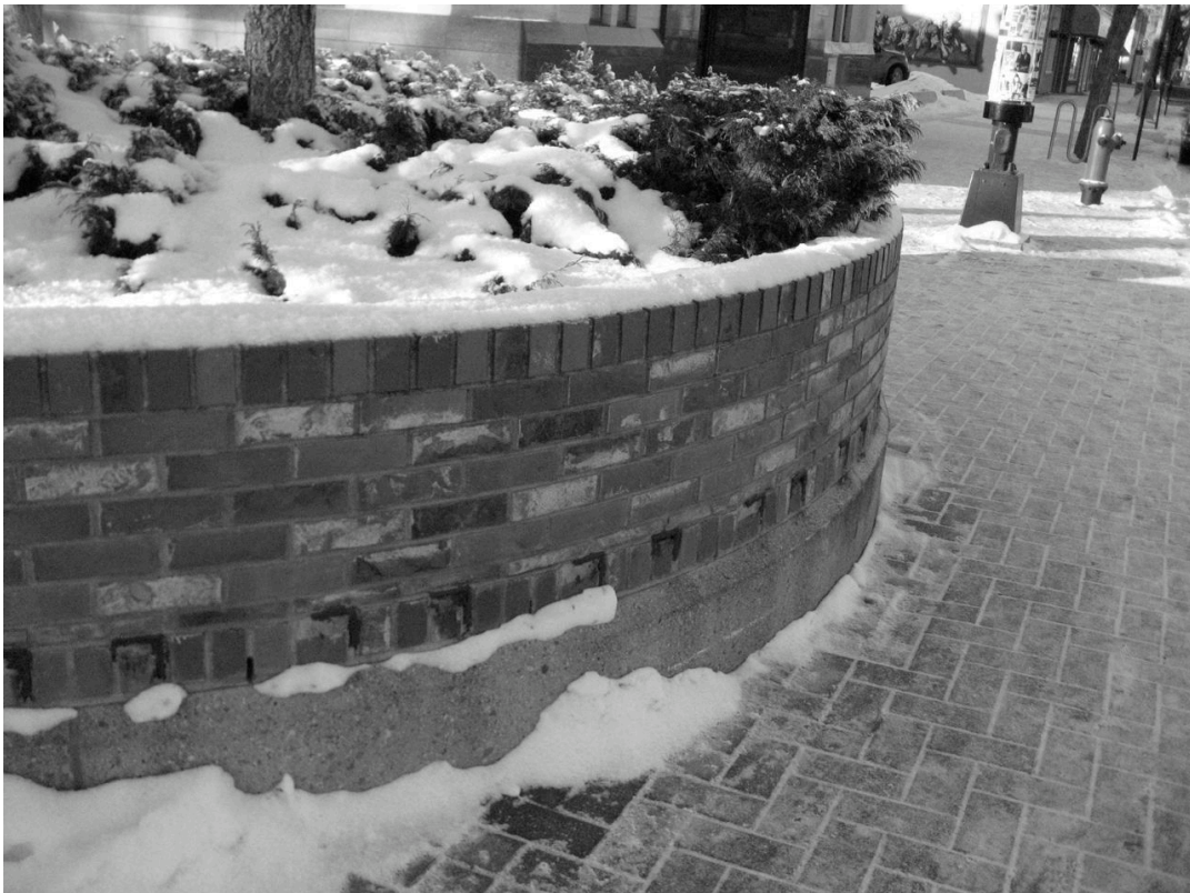
Figure 1. Skeleton of sawed-off public bench across the street from Galt Gardens.
