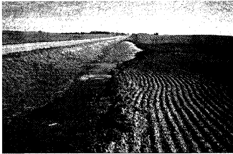
Figure 16 Road induced runoff accumulation
