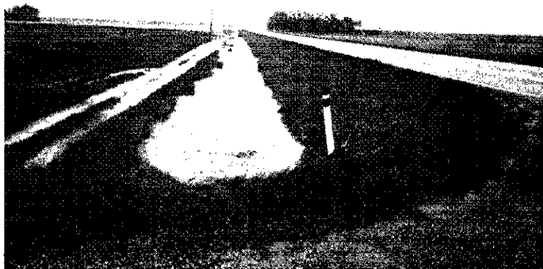
Figure 14 Road induced runoff flow path modification
