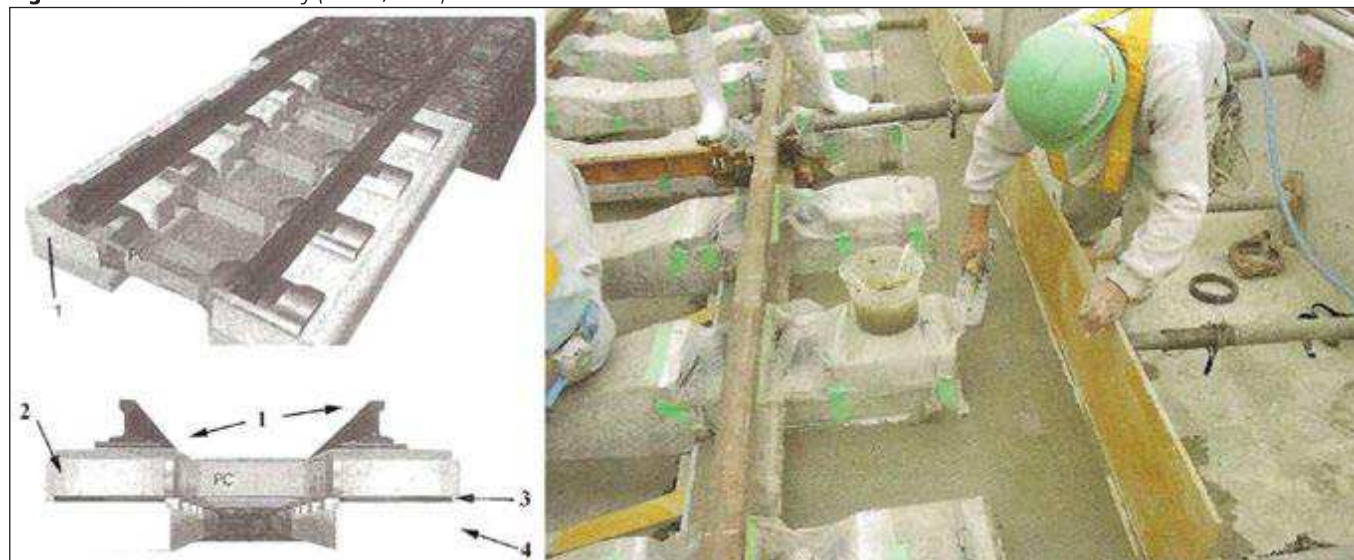
Fig 1: Elasto Ballast track railway (Ridout, 2009)
