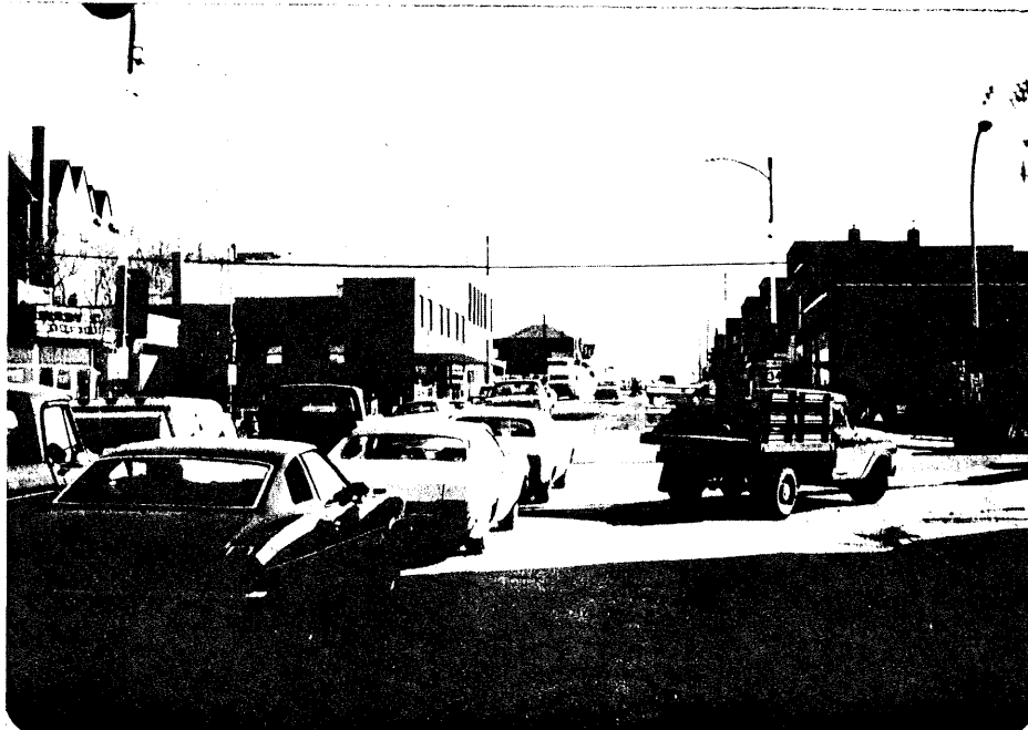
Looking east at the nonconforming Main Street signals.
