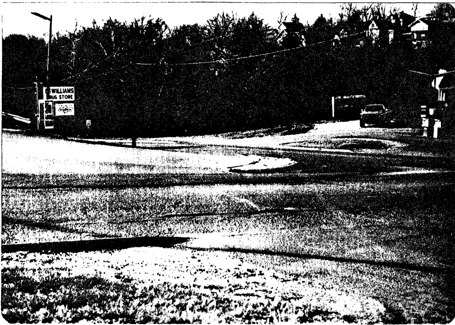
The southeast corner of Pennsylvania and Jefferson as seen from Pennsylvania Avenue.
