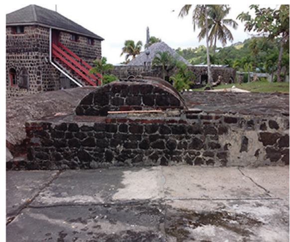
FIGURE 2 | Brick vaulted cistern and casemate structure, Old Fort, Bequia, St Vincent Grenadines (plan and elevations; scale at right in photograph 1 m).
