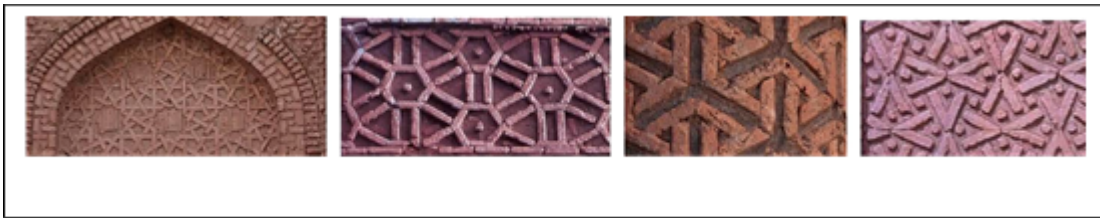
Figure 32. Tower of Kharraqan in Qazvin, 12-point, 6-point, abstract 6-point, and 8-point geometrical patterns. (From Abdullahi, 2013.)
