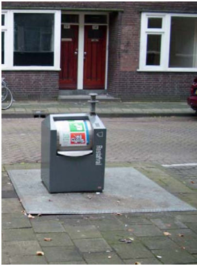
Figure 1. Underground garbage container
