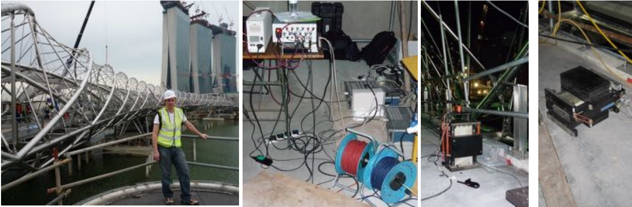
Figure 1 Modal test of Helix Bridge, Singapore using two shakers
