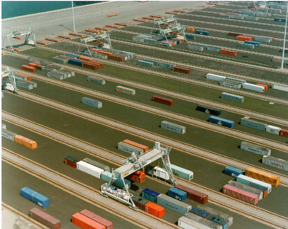
Figure 3.2: Stack lanes with ASCs (photo: courtesy of ECT)
