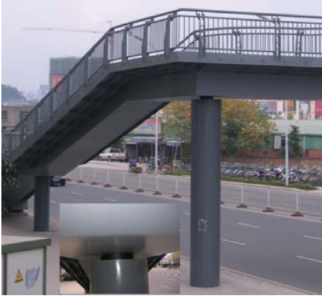
FIGURE 1: CFST column subjected to partial compression [4].
