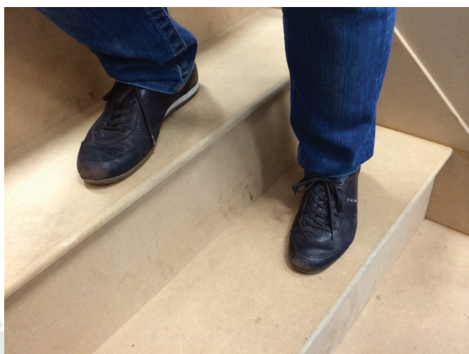
Figure 2. Foot positioning during descent in a staircase with 175 mm rise and 310 mm going (top), and in a staircase with 220 mm rise and 220 mm going (middle and bottom). In the 170 mm-rise and 310 mm-going configuration descent the feet look forward and there is enough room to place the ball of the lead foot within the step (top). In the 220 mm-rise and 220 mm-going configuration, if the feet are placed forward, the ball of the lead foot is placed outside the edge of the step, which can reduce balance and result in a fall. Sideways placement of the feet (bottom) circumvents this problem.
