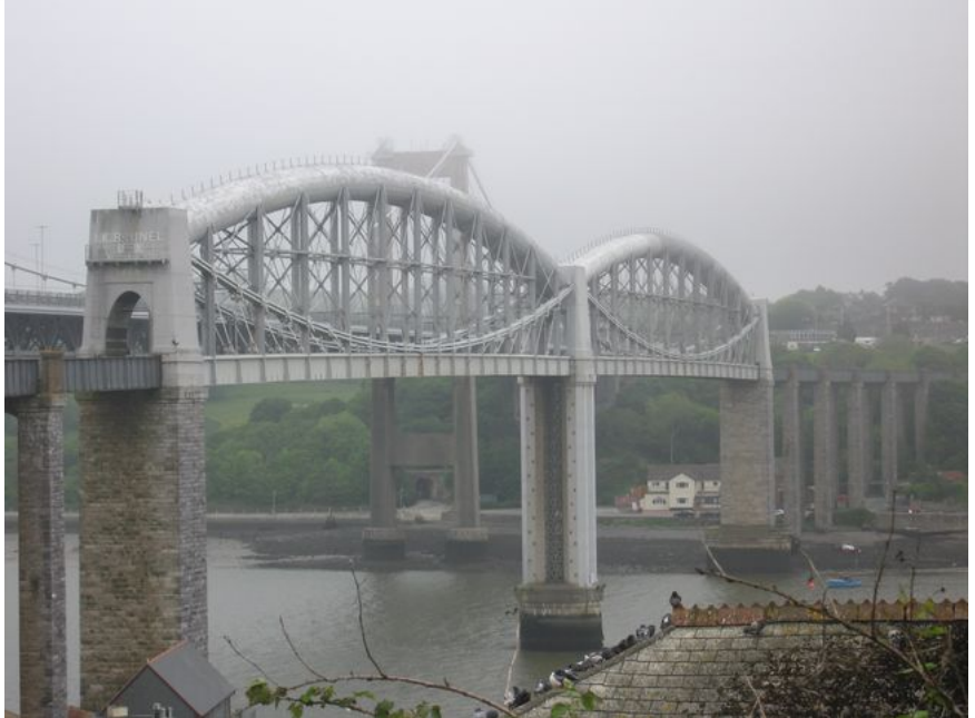
Royal Albert Bridge at Saltash
