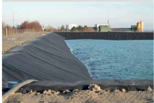
Figure 37 75000 m 3 water pond under construction at Marstal solar heating plant.
