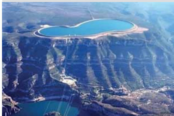
Figure 12 Pumped hydro storage facility in Spain illustrating the topographical requirements for traditional PHS installations [9].
