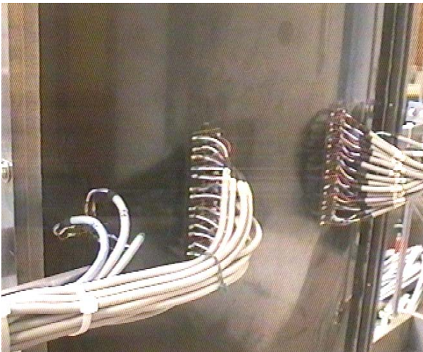
FIGURE 9. Panel with strain-gauges
