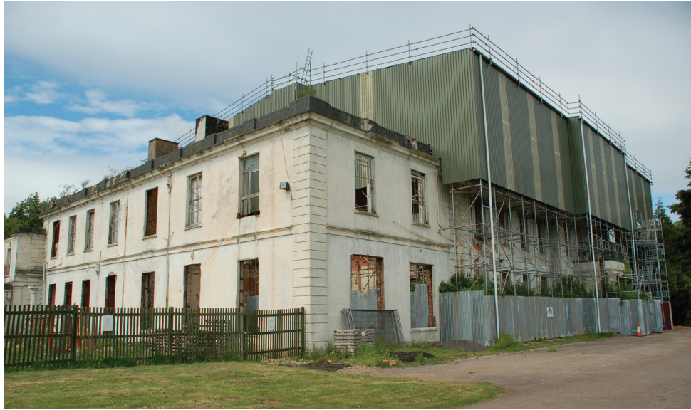
Plate 1. View of Poltimore House from the south-west, showing the roofless ballroom to the left and the early eighteenth-century frontage to the right, obscured behind a temporary corrugated iron roof installed to protect the property from further damage (Photograph: Oliver Creighton).
