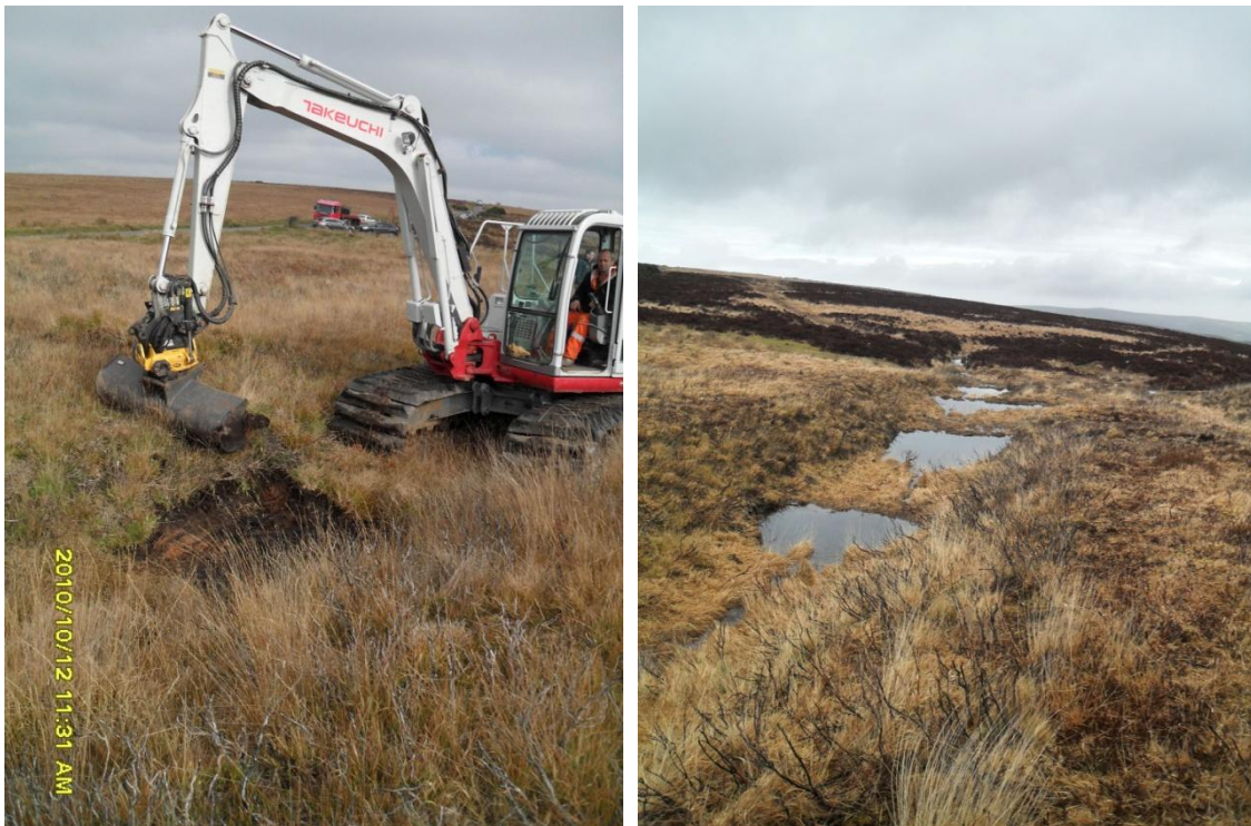
Fig. 6.3 Upland ditch blocking undertaken by the National Trust in the upper reaches of the Horner Water catchment between 8 th September and 14 th October 2011 with the aim of increasing water storage and reducing the velocity and magnitude of discharge response to rainfall events.
