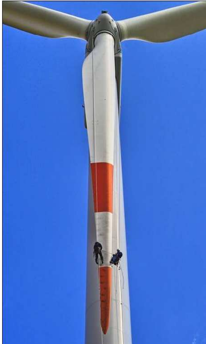
Figure 1.8: Repairs of wind turbines at Windpark Prettin, GE Energy, Saxony-Anhalt [21].
