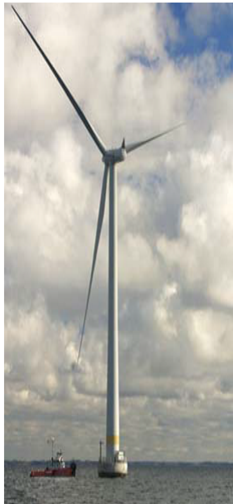
Figure 4.30: The picture shows a Siemens SWT-2.3-93 in Lillgrund [90].
