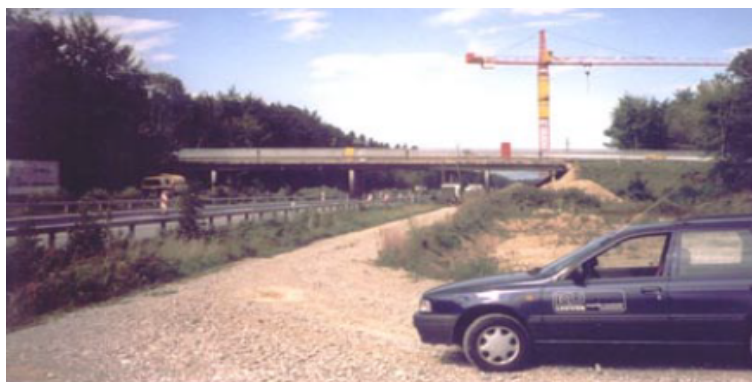
Figure 6.1: View of Z24 Bridge.
