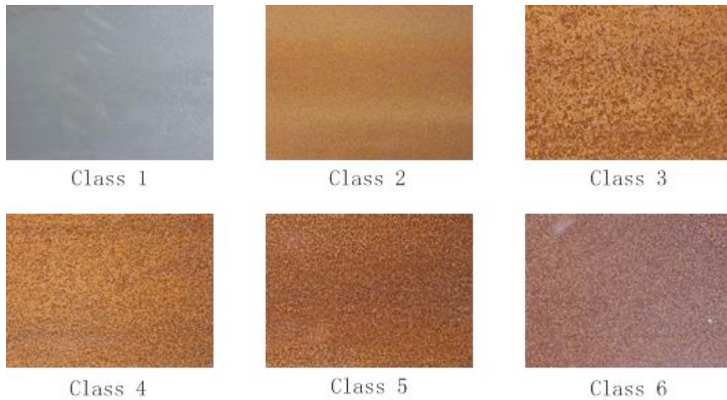
Figure 3.5 One set of rust images which contains six classes
