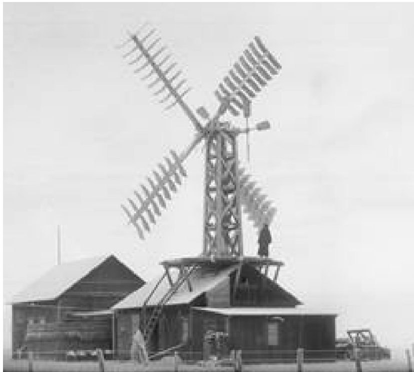
Figure 1.2: Poul LaCour's turbine: the beginning of the wind energy industry in Denmark (Askov Laboratory, 1891), reproduced from [1].
