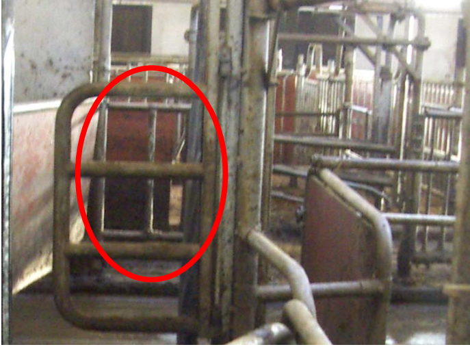
Picture 6. In the red oval one can see the hole between the pipes, where cows used to put their head from the feeding table side and keep other cows from walking through gate 2 to the feeding table. This also gave false registrations in gate 2. On March 14th a board was put in this place to get rid of the problem and it has helped a lot. Cows walking through gate 2 no longer hesitate as much as before.
