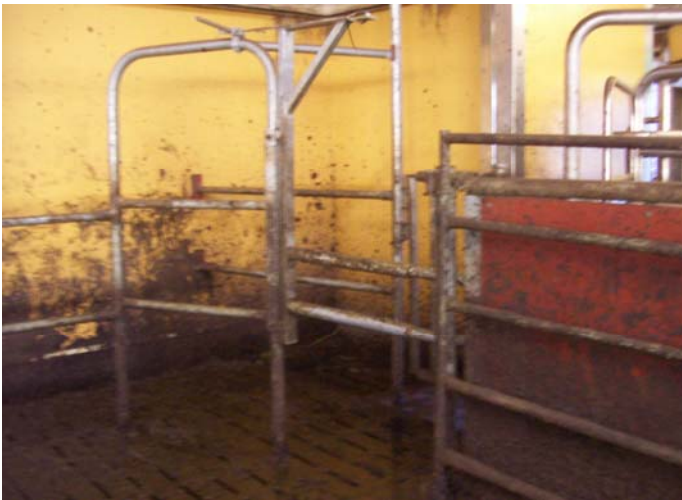
Picture 3. The end of the precedence passage, view from the waiting area. In the middle of the picture one can see the push gate which separates the precedence cows from the waiting area cows. To the right is MS2. In and around the precedence passage there is slatted floor.
