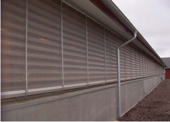
Picture 10. DeBoer Ventilation at Farm A. When it gets to warm in the barn, the walls are automatically let down to let more air in. This is combined with natural ventilation through the roof ridge.
