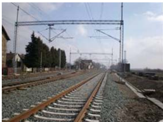
Section of reconstructed railway
