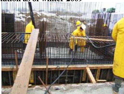
Pouring concrete foundations
