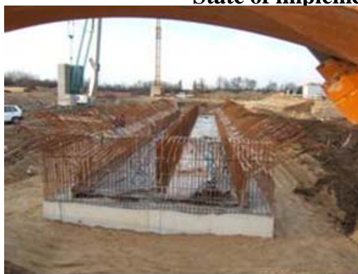
Construction of foundations
