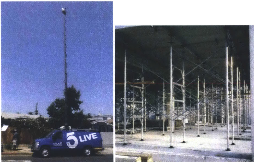
Figure 2 - Left: telescoping antenna on a news van. Right: adjustable height construction shoring
