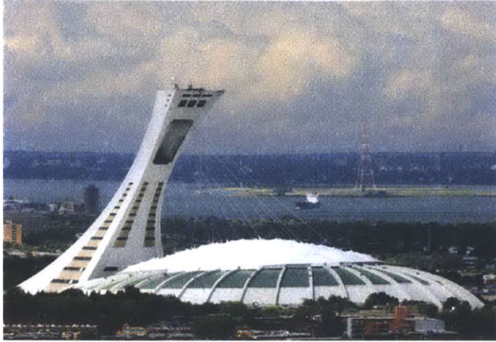
Figure 6 - Deployable roof on Montreal's Olympic Stadium, designed to be retracted with cables
