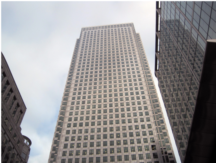
Figure 8-3 High-rise buildings in Canary Wharf (Source: Author)
