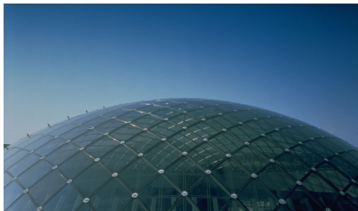
Figure 1.7: Roof of a swimming pool in Neckarsulm ( photo: www.sbp.de )
