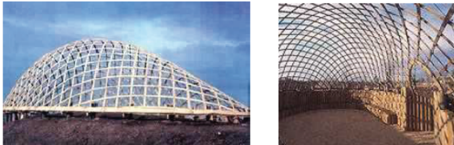
Figure A.5: Earth Centre grid shell
