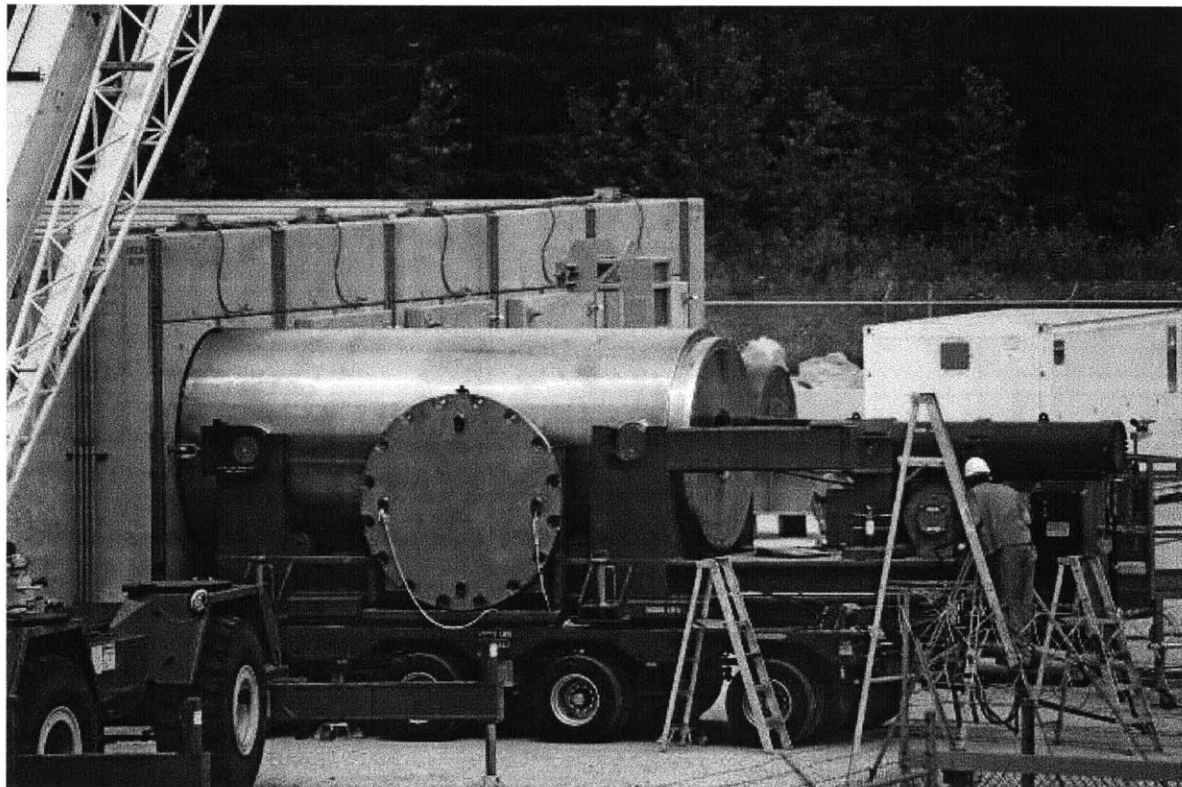
Figure B.3 - Dominion Test Run of a NUHOMS canister transfer from TC to HSM [Content, 2013]
