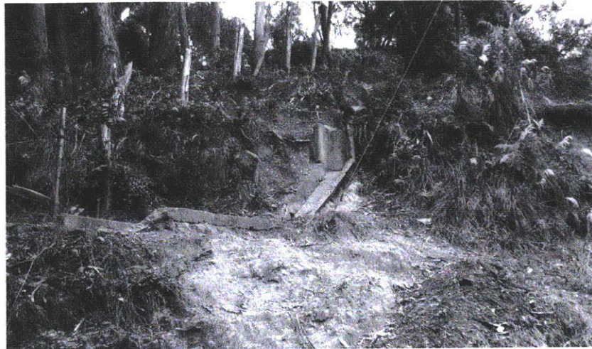
Fig 4.09 Makeshift Canal Photograph of makeshift water infrastructure in an informal settlement and erosion around it.
