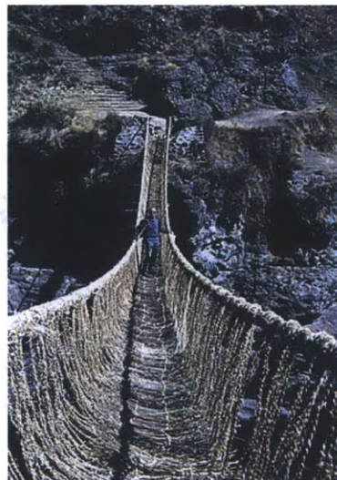
Figure 1: Inca rope bridge 3
