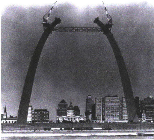
FIG 13: St. Louis' Gateway Arch under construction
