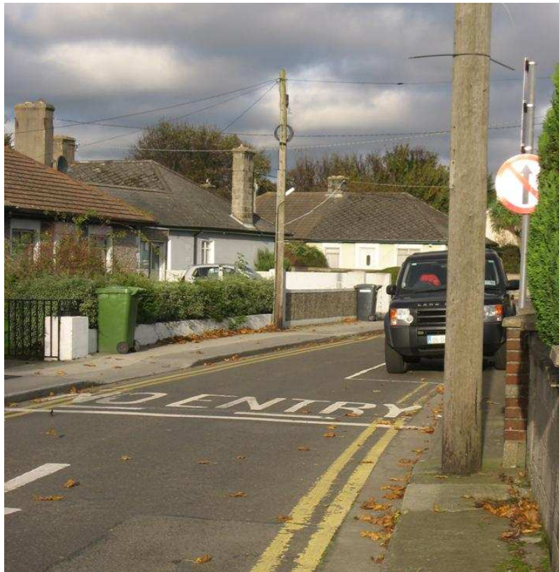
Figure 4-11: Narrow footpaths as a result of meeting highway design standards
