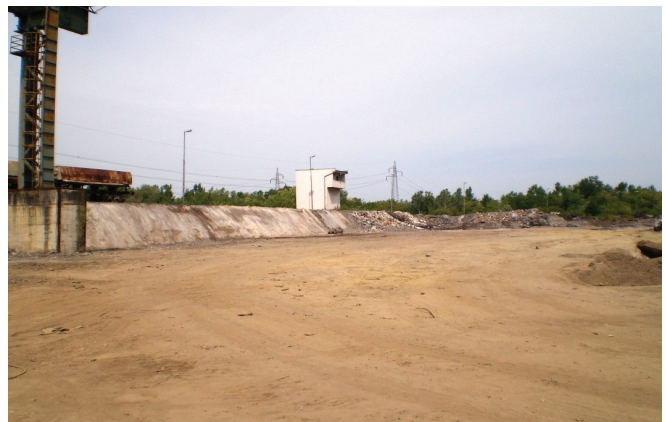
Fig. 2 – Landfill after cleaning and removal of waste
