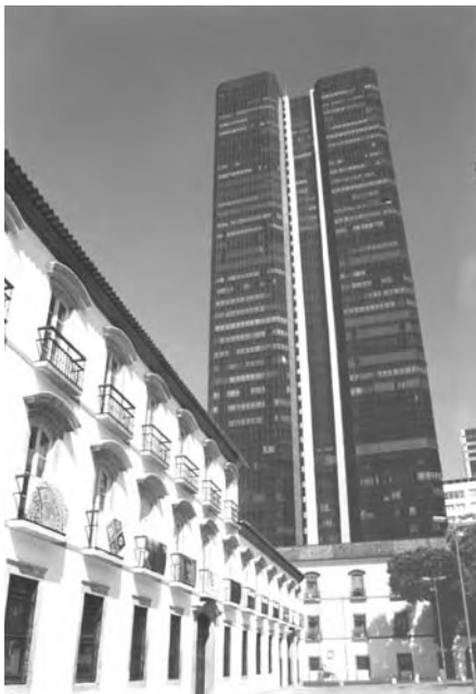
Contrast between a historical building turned museum and a modernist skyscraper. (Photo: V. del Rio)
