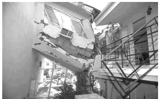
Destruction by the Northridge earthquake in Los Angeles, 1994. (Photo: OES, California)
