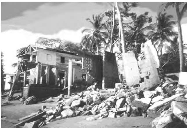
Damages on Honduras South Coast, Hurricane Mitch, 1998. (Photo: OES, California)
