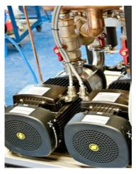
Figure 4. Redundant Pumps in CDU
