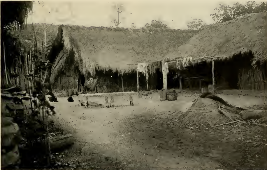
From this compound, at the very edge of a central Hainan forest, pioneering Cantonese manage one of their new tobacco plantations. Kang, one of the "taxidermists" of the expedition, made the compound his headquarters for many days. These thatched houses, with walls made of upright saplings, are the coolest and most economical houses that can be built. The compound is protected by a living stockade. In the center of the picture a few skins may be seen sunning
