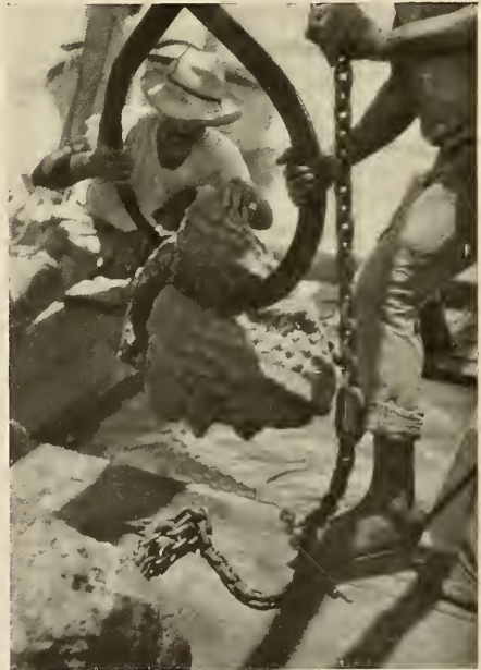
Raising a coral specimen to the deck of the pontoon by means of steel tongs and a ten-ton chain hoist. Though very heavy specimens were successfully lifted in this way, the tough steel of the tongs was finally bent in an endeavor to secure an unusually large example
