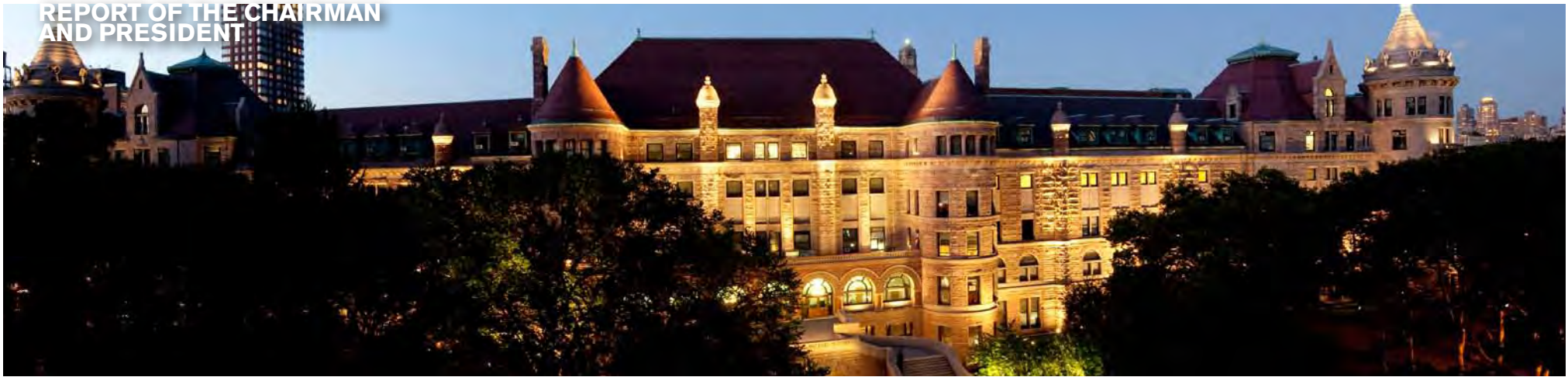
The renovated 77th Street façade features a new exterior lighting scheme.
