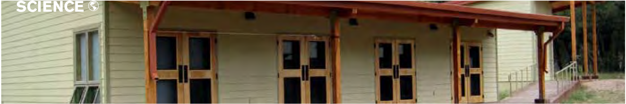
The new Education Building of the Southwestern Research Station near Portal, Arizona, was completed in fiscal 2009.
