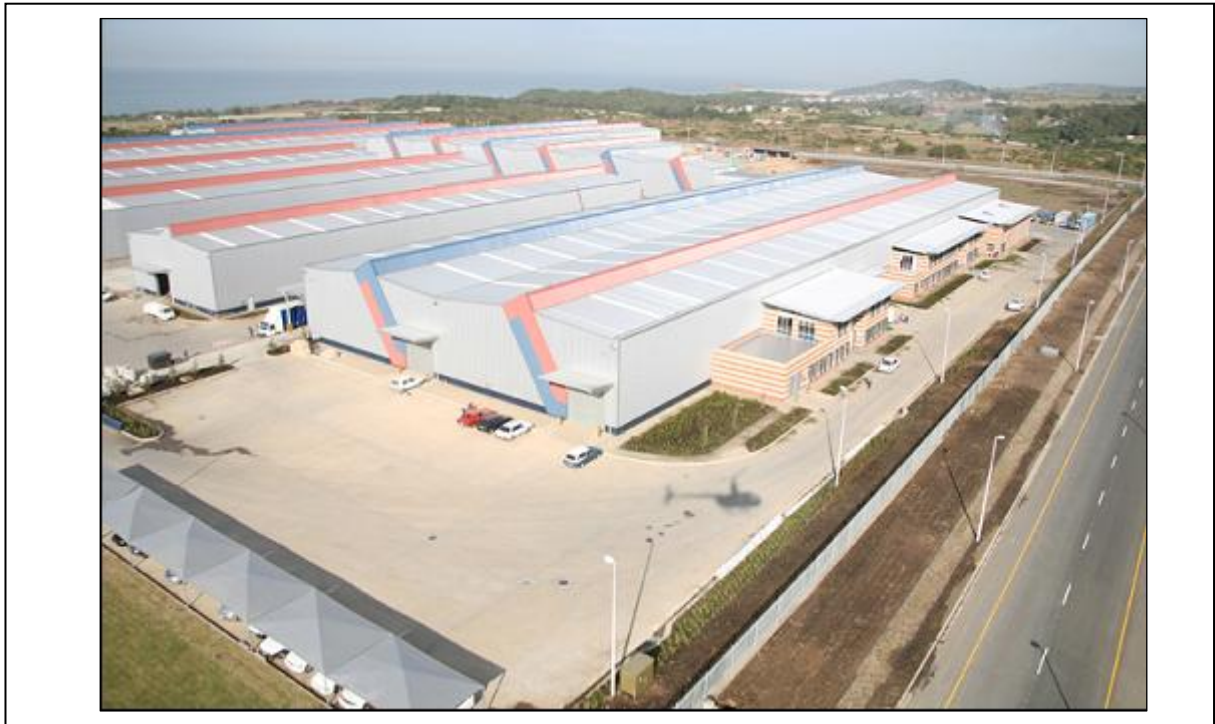
Figure 5.6 – An aerial view of one section of the East London industrial development zone
