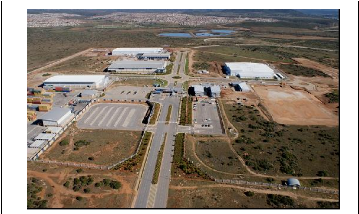
Figure 5.7 – An aerial view of the Nelson Mandela Bay logistics park
