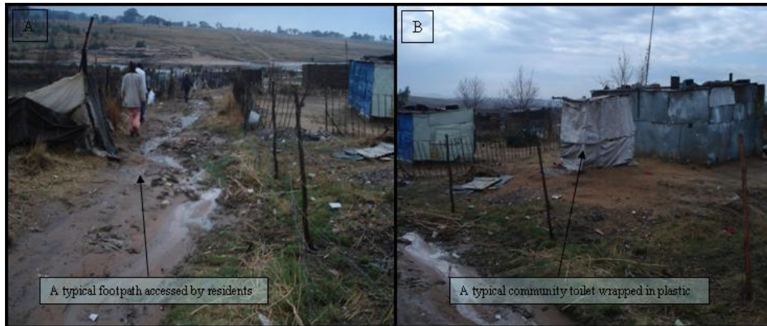
Figure 18: Eroded footpath leading to other dwellings affected by heavy rains
