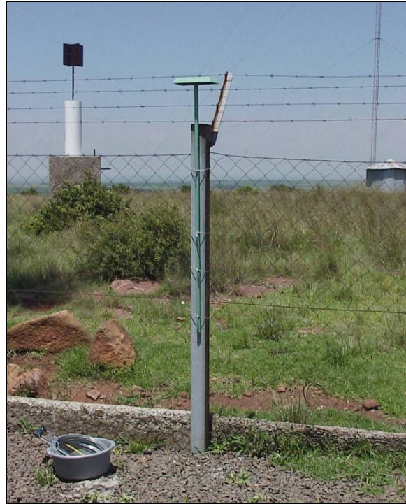
Figure 2.2: A passive sampling monitor in position (Sampling site no. 17, Elandsfontein).
