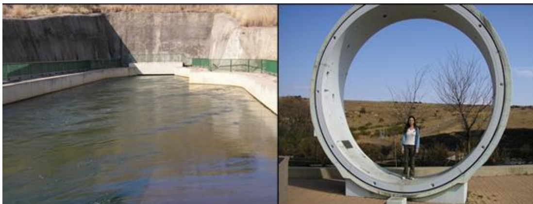
Figure 4: Ash River outfall tunnel (left) and water delivery pipe size (right).
