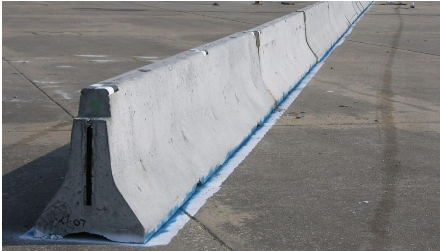
a) Free-Standing Temporary Concrete Barriers
