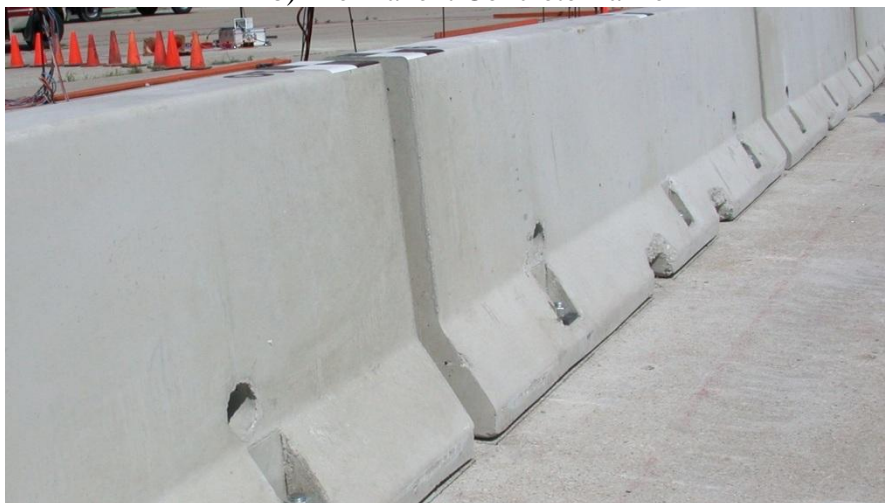
c) Temporary Concrete Barriers with Restrained Movement
