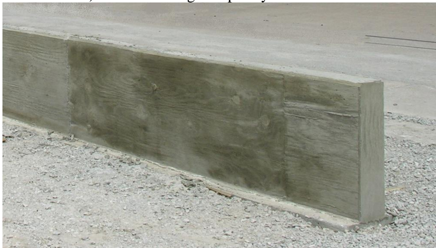
b) Permanent Concrete Barrier
