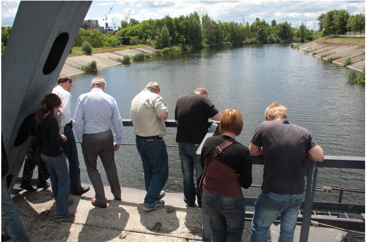
Image 66: Feeding the catfish. The rusting hulks of the half-built reactors 5 & 6 with still standing cranes can be seen in the background. (#p0633)
