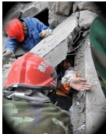
Figure 2.1: An example of a life safe void
