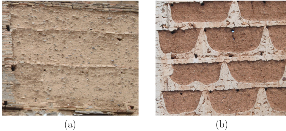
Figure 1.1: Examples of RE construction variations (Villafeliche, Zaragoza, Spain, c. 12 th century): a) use of brickwork ( chained RE) ; b) use of lunetos . Photographs by Paul A. Jaquin. Used with permission.
