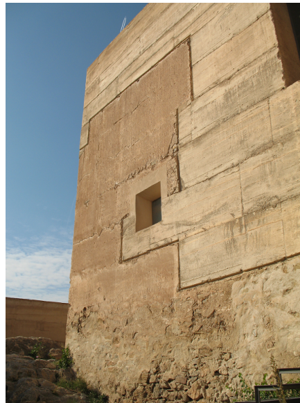
Figure 8.4: Earthen repairs made to Castillo Cox, Valencia. Photograph by Paul A. Jaquin. Used with permission.
