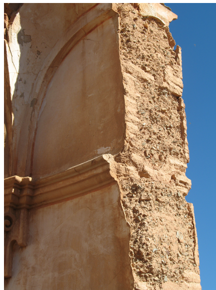
Figure 8.2: Moulding of earthen render in Villafeliche, Zaragoza. Photographs by Paul A. Jaquin. Used with permission.
