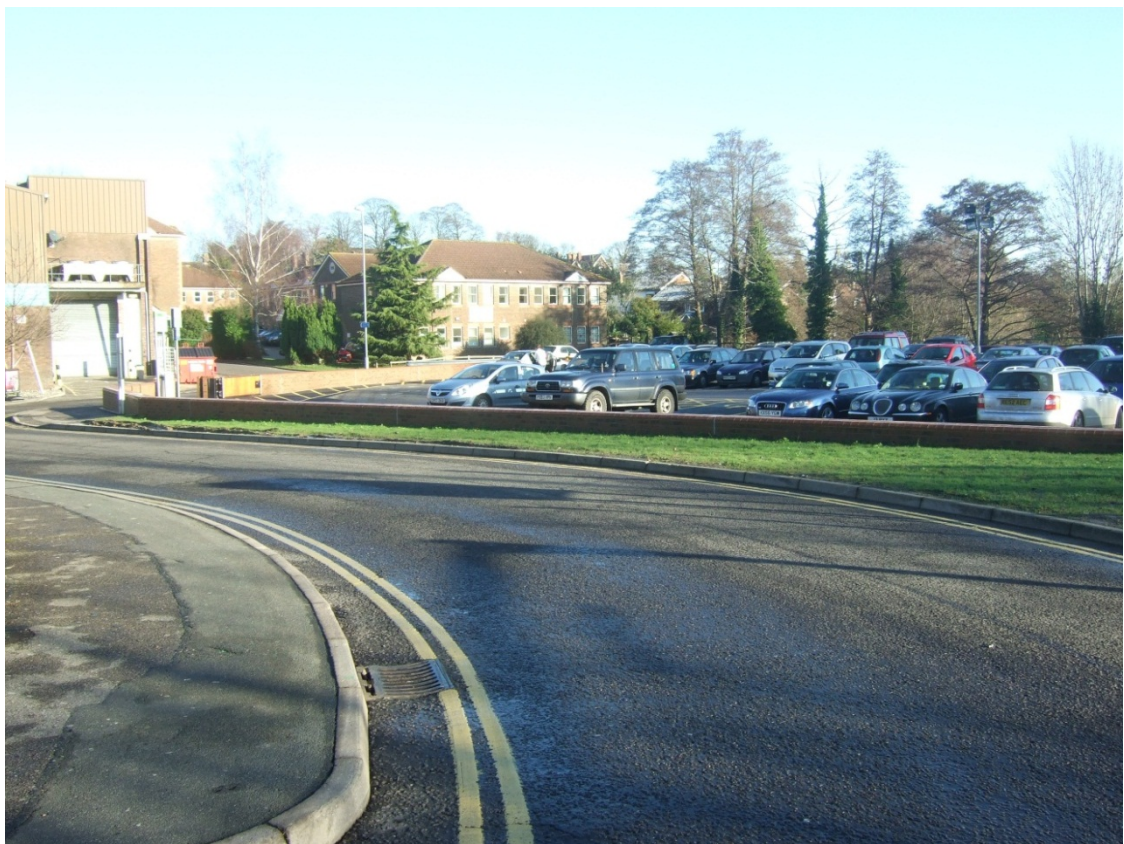
Figure 3.6. Uckfield flood wall, facing roughly east
