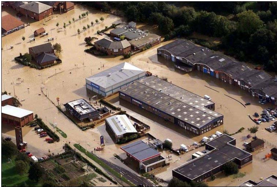
Figure 3.3. (BBC, 2009) Flooding in Uckfield, October 2000
