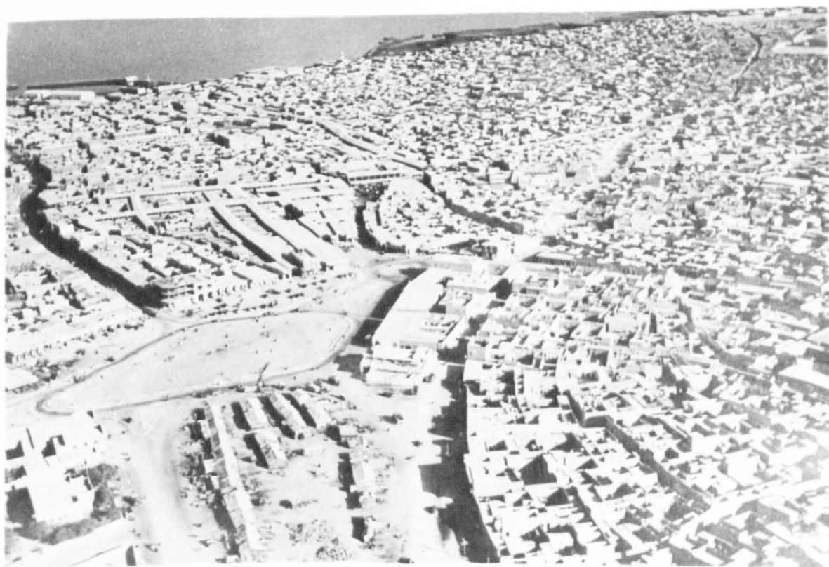
Plate 7.2 Safat Square and the Suq looking northwards about 1940.
