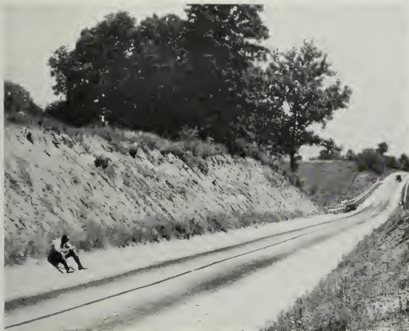
FIG. 5a.—Exposure showing a two-cycle weathered profile on glacial drift beneath loess, resulting from dissection after development of the gumbotil and before deposition of the loess. One mile east of Trenton, Illinois, east-central part of Sec. 21, T. 2 N., R. 5 W., Clinton County (photo by MacClintock).
