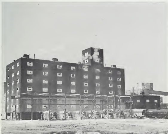
Figure 14 - View of Olin Mathieson Chemical Corporation's hydrofluoric acid plant at Joliet, Illinois. Note the six rotary kilns in lower foreground. (Photograph courtesy of Olin Mathieson Chemical Corp.)
