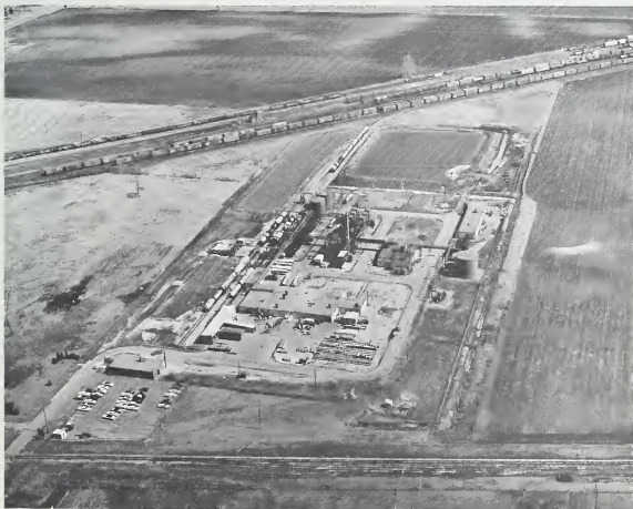
Figure 15 - Aerial view of the Genetron fluorocarbon plant of General Chemical Co. - Division of Allied Chemical Corporation near Danville, Illinois. (Photograph courtesy of Allied Chemical Corp.)
