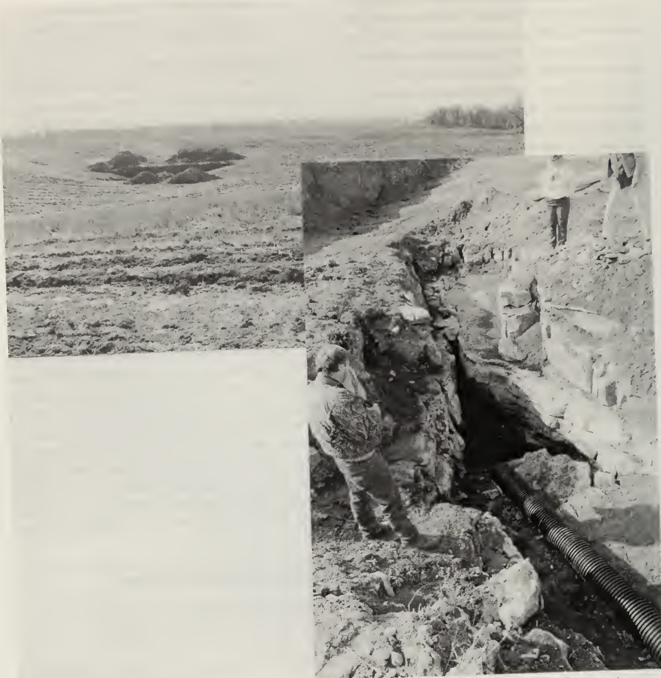
Figure 27. An excavated sinkhole revealed a long crevice in the exposed bedrock that leads to a somewhat wider crevice. The crevice led down, about 15 feet, into a small cave about 1 foot high and 2 feet wide through which rainwater and snow melt flowed.
